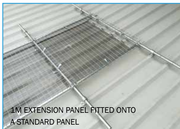
BASE FITTED ONTO ROOF PANEL
