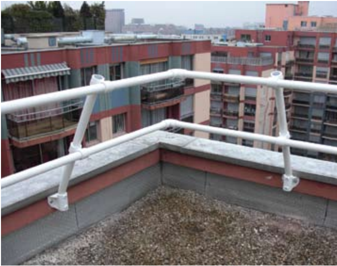
Kee Modules® side fix mounted, handrail tube in-line
