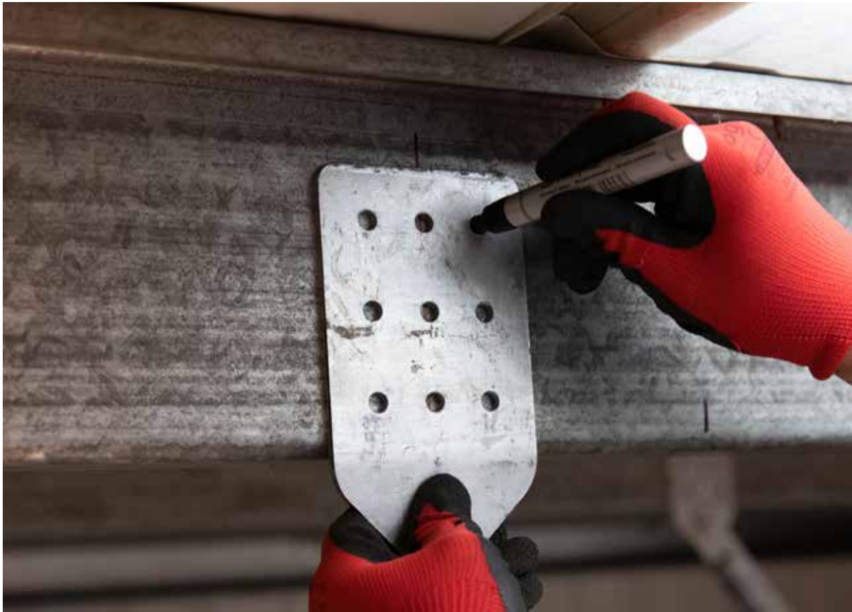
Fig. 1: Incorrect - bracket bends towards you
