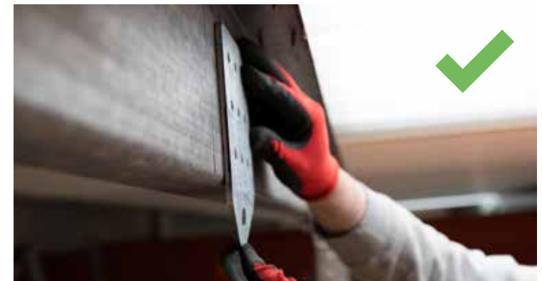
Fig. 2: Correct - bracket bends away from you
