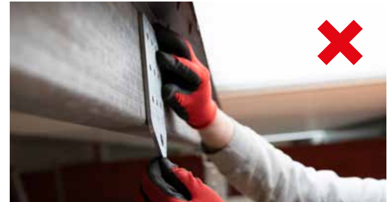
Fig. 1: Incorrect - bracket bends towards you
