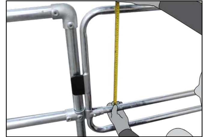
Q. Use a measuring tape to ensure gap between top rail and mid rail is no more than 470mm. Adjust if necessary.
