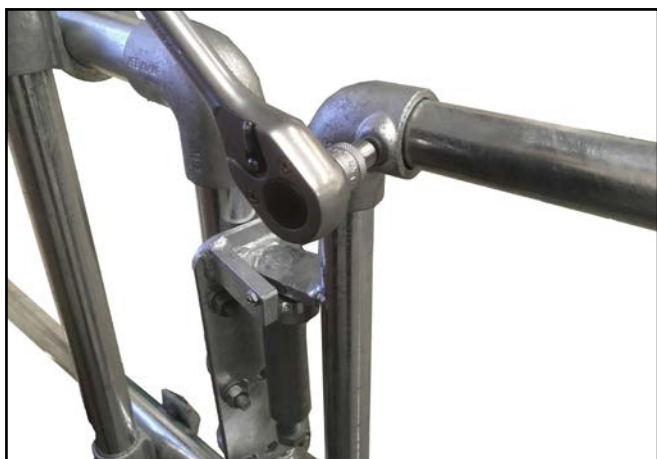
I. Carefully re-position the gate top and bottom tubes into the cast fittings. Use a spirit level, to ensure the gate is level. Tighten the cast fittings grub screws using a hex head socket. Using the torque wrench ensure the castings are torqued to 39Nm.
