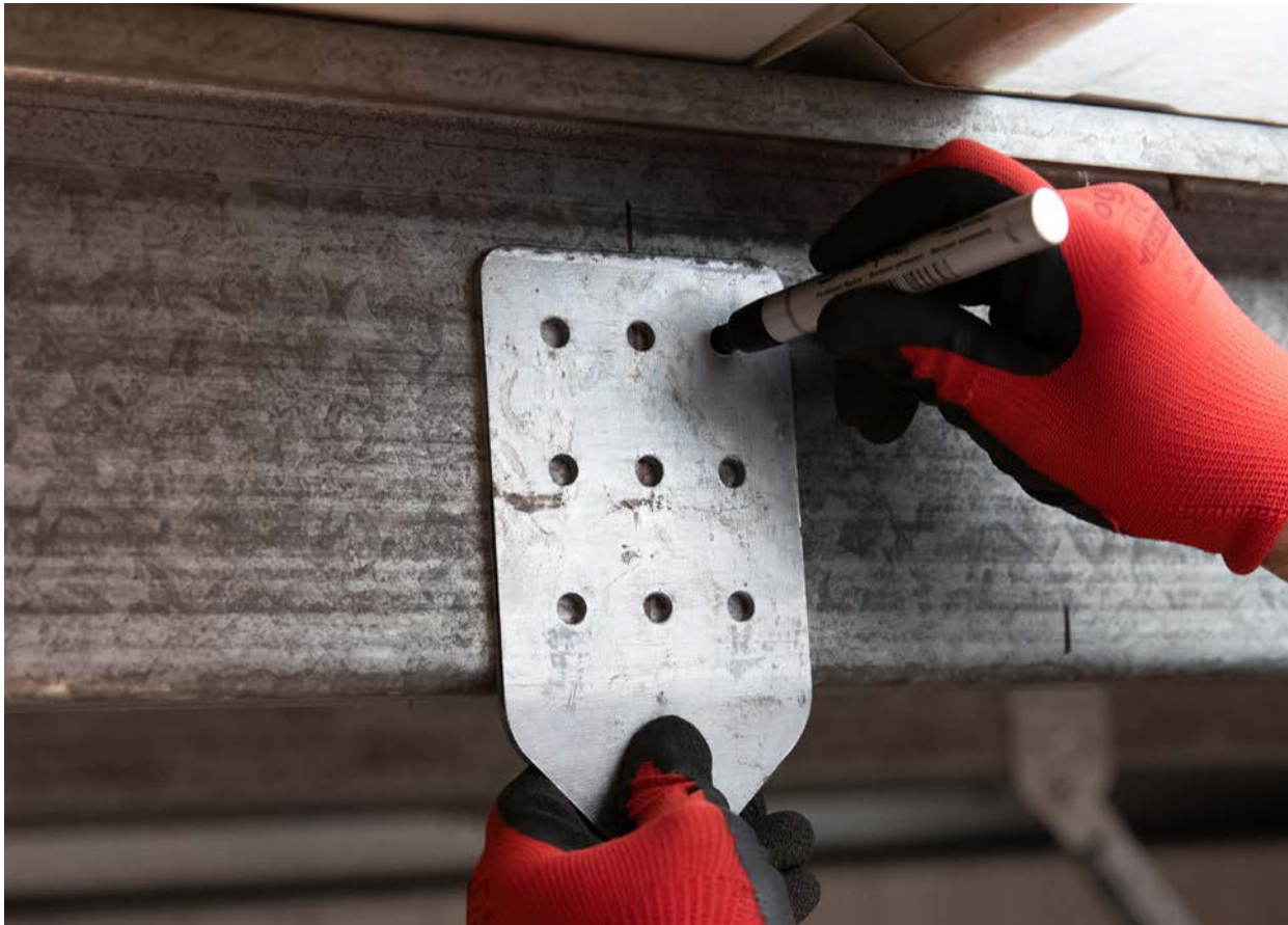
Fig. 1: Incorrect - bracket bends towards you
