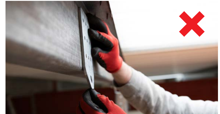
Fig. 1: Incorrect - bracket bends towards you
