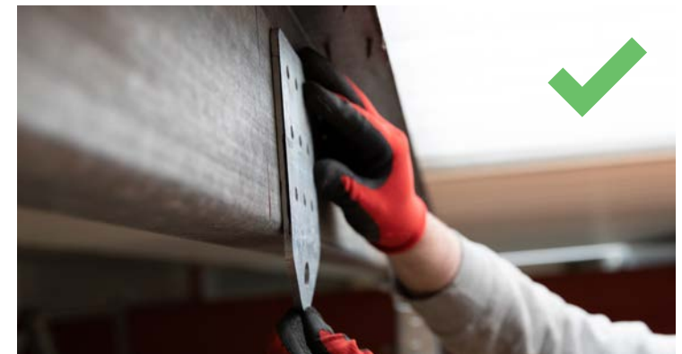
Fig. 2: Correct - bracket bends away from you
