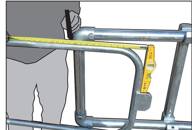
F. To cut the gate to the correct size simply place a straight edge/magnetic level as shown and measure the distance to the point where the outside edge of the vertical tube meets the supporting structure as shown. **(DO NOT CUT AT THIS MARK!)**
