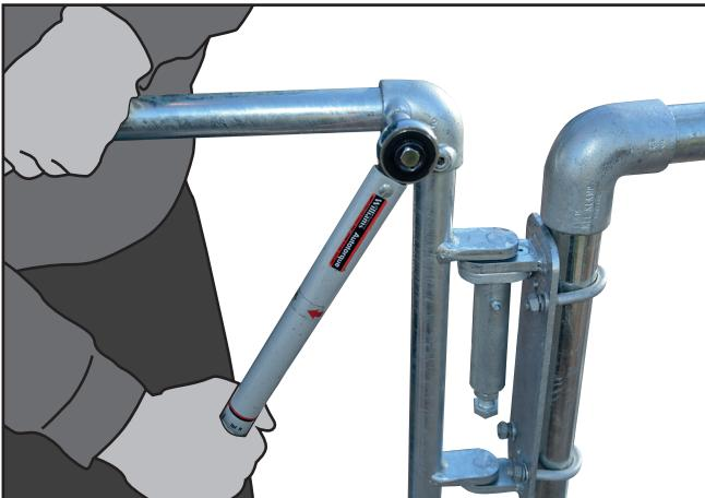
**GB** - J. Carefully re-position the gate top and bottom tubes into the cast fittings. Ensure the striking plate is on the correct side of the Support Leg/Structure. Use a spirit level, to ensure the gate is level. Tighten the cast fittings grub screws using a hex head socket. Using the torque wrench ensure the castings are torqued to 39Nm.
