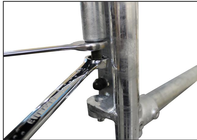
**GB** - M. Using the 24mm socket & ring spanner start to tighten the bolt until the gate completely closes. (Note:- You may have to hold the socket whilst using the ratchet).
