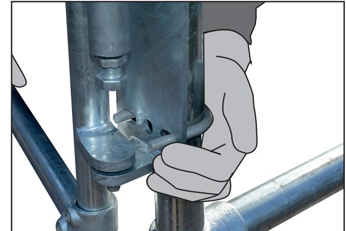
**GB** - A. Align the fixing plate on internal face of the opening, so that the rails of the Safety Gate match up with the top of the Guardrail System. Select the correct U Bolt & pass it through the Steel Safety Clamp & around the support leg/structure and feed through the top holes of the fixing plate.
