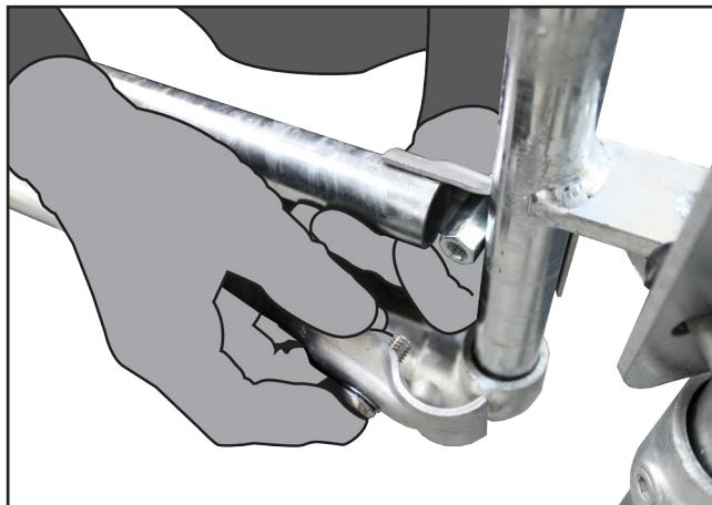
P. Add clamp onto other end of mid rail, clamping onto the gate upright. Use 6mm hex head socket to tighten supplied M10 bolts into coupling nut. Using the torque wrench ensure the clamps are torqued to 20Nm.
