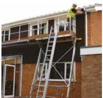
Two or more Easi-Dec platforms can be securely linked with our Catwalk to provide a continuous fully guarded platform compliant with edge protection requirements set out in EN13374.
