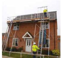
The Solar Access System provides a safe working platform combined with certified edge protection at roof level. The system comprises one Solar Platform, one Easi-Dec platform and a Catwalk which provides either an 8m or 10m long working area. Additional Decs and Catwalks can be added to provide a limitless modular system.
