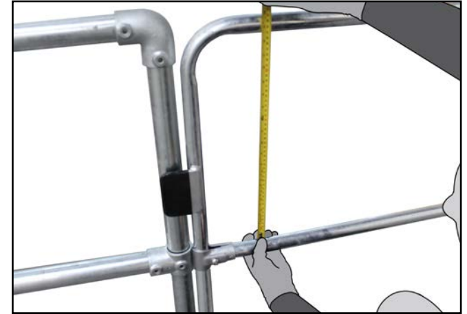
N. Use a measuring tape to ensure gap between top rail and mid rail is no more than 470mm. Adjust if necessary.
